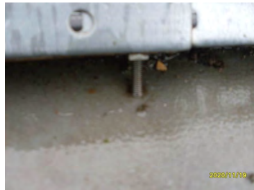
Screw from tray touching the membrane
