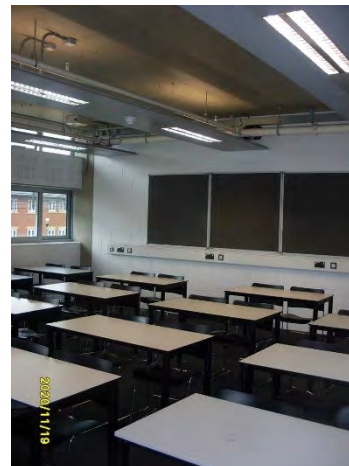
Typical classroom view
