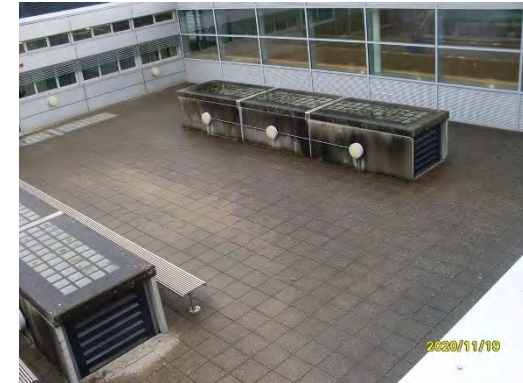
Concrete enclosures due for cleaning
