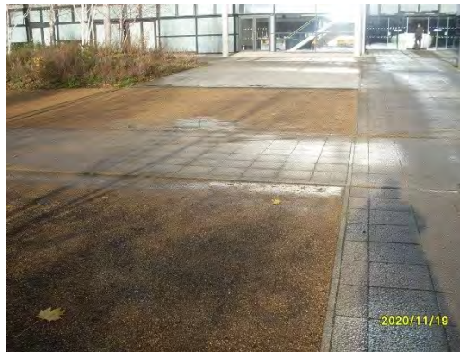
Compacted gravel paving
